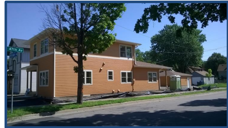
2 ADUs (+ 2 under construction)
